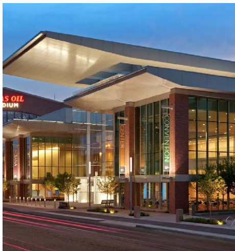
Site of the Church of God 79th International General Assembly— Indiana Convention Center, Indianapolis, Indiana
